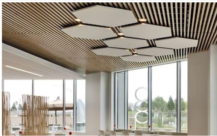
Aluminum Strips Ceiling
